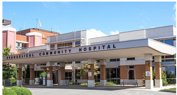
Evangelical Community Hospital Lewisburg, PA
