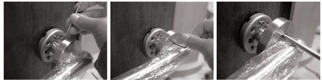
Use allen wrench in between rose cover and under-construction.
